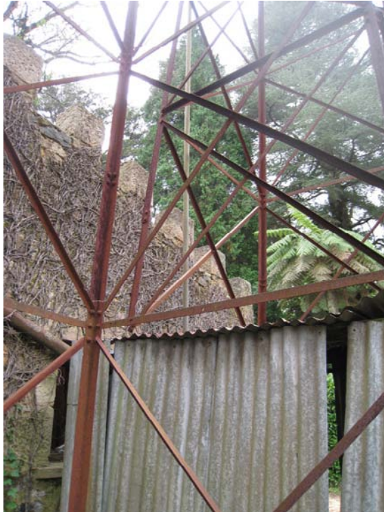
Figure 15: Detail of the framing.
