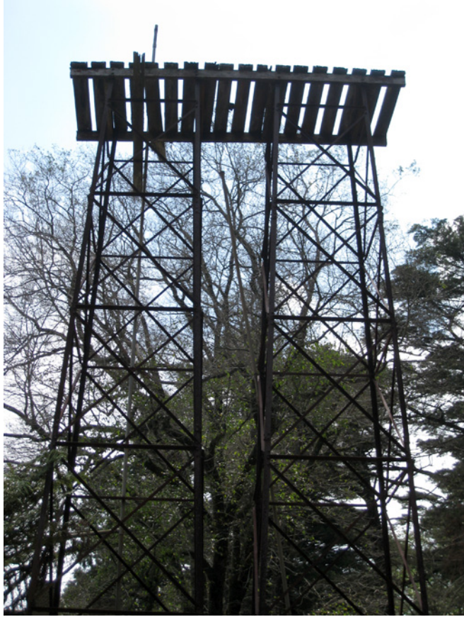
Figure 13: Timber platform at the top of the water tank stands.
