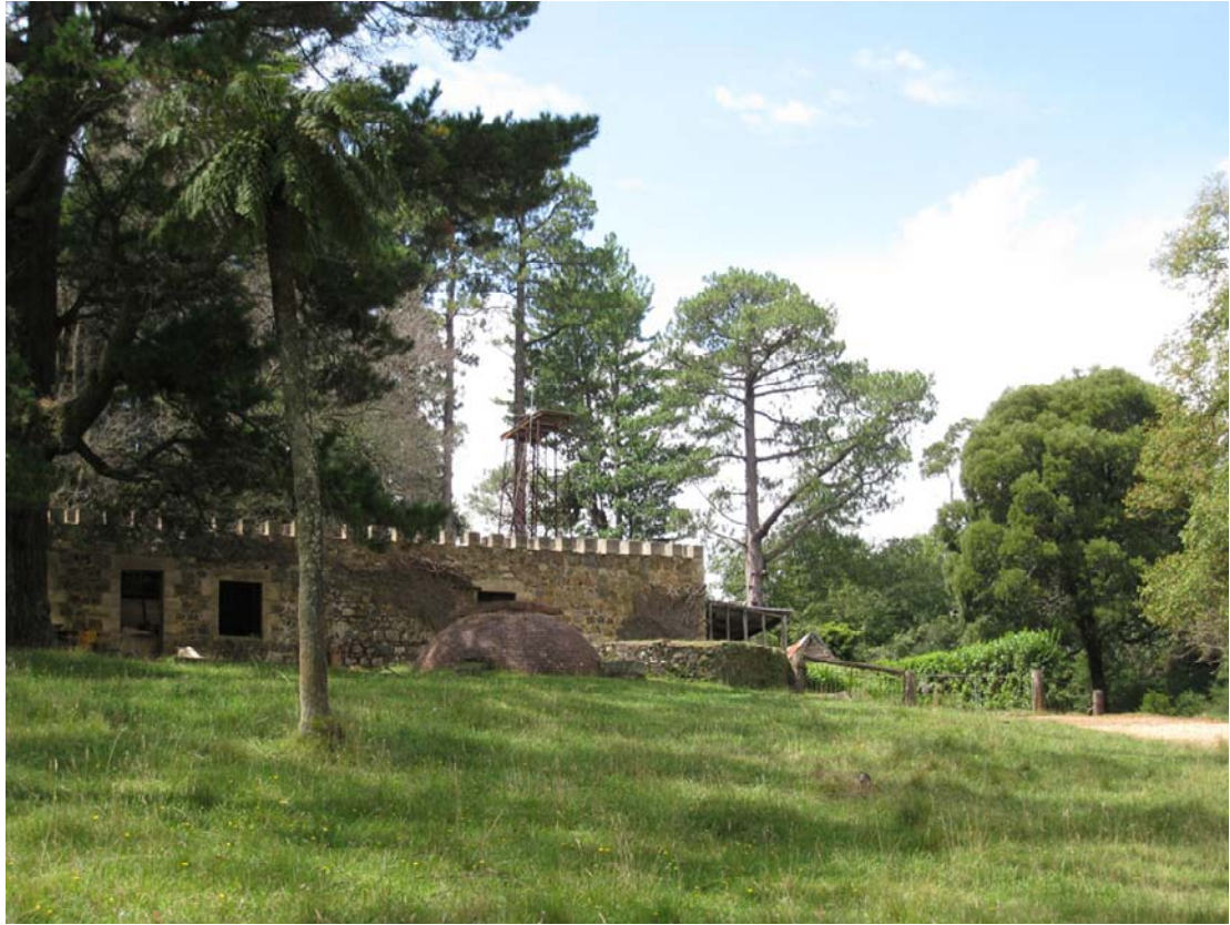
Figure 1: Approach from the driveway, looking east. The water tank stands can be seen behind the Stables
