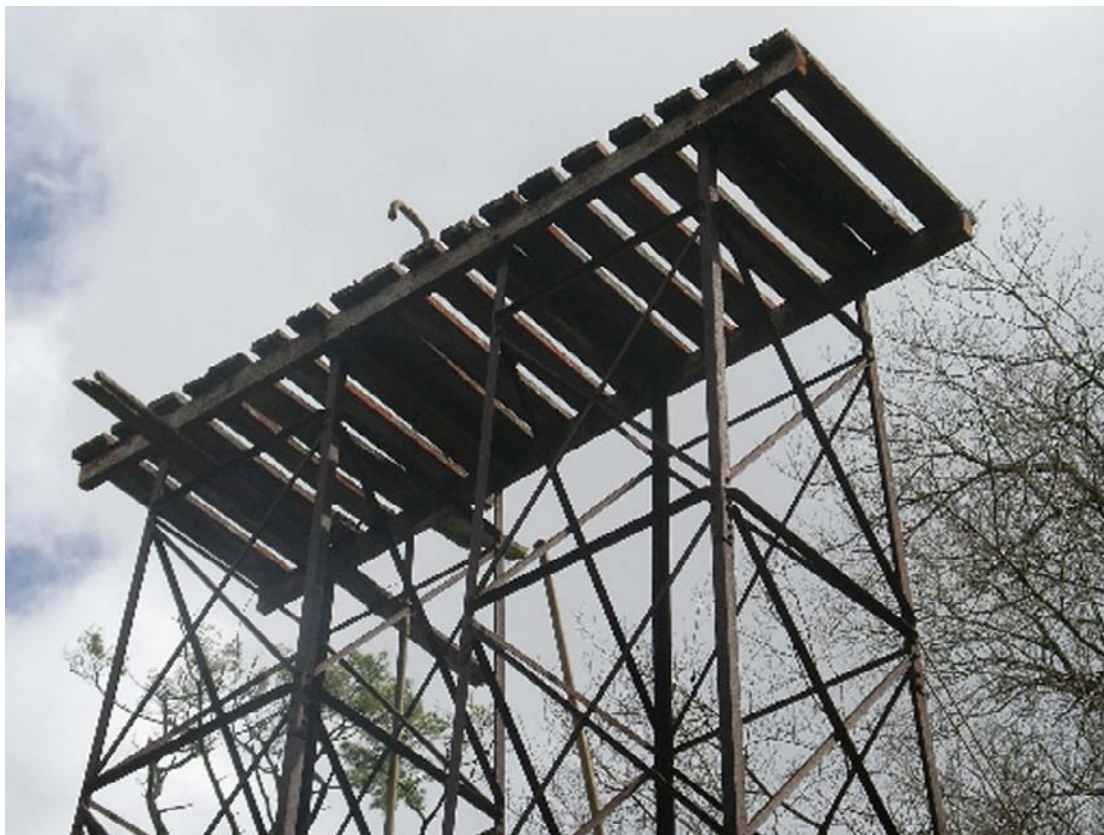
Figure 14: Timber platform at the top of the water tank stands.
