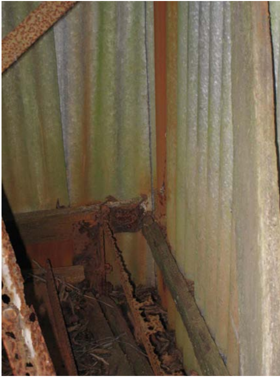
Figure 19: Detail of the framing.
