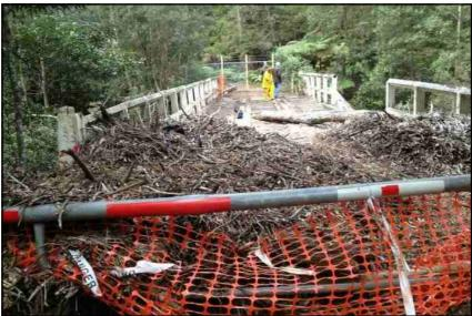
The bridge is fenced off in both directions, guard railings have broken away and mounds of debris from the flooding creek cover what was once a road.
